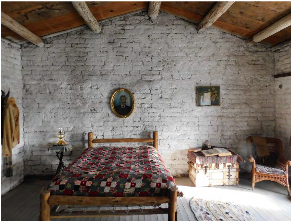
View looking North; the adobe has been whitewashed in a manner that is described in early written descriptions.
