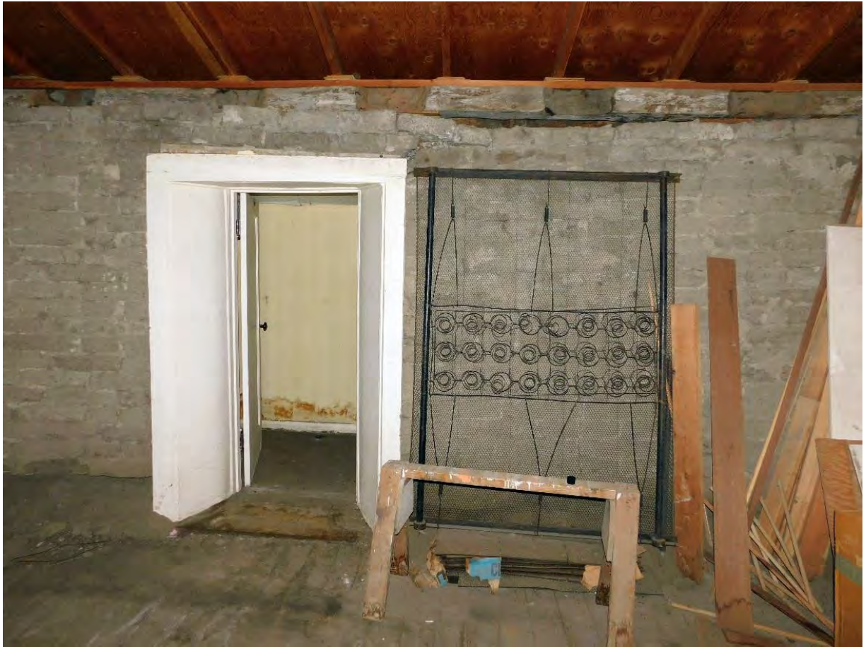
View of West Wall; note wood infill at top of original adobe on the right side of the door.
