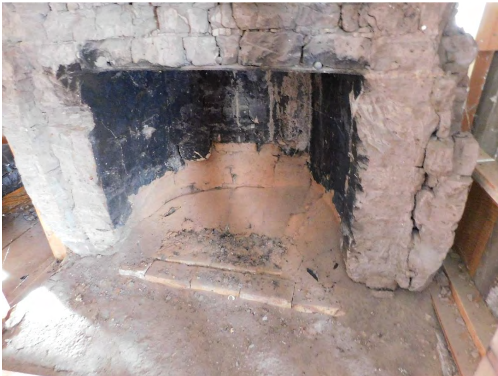
Fireplace in Room 103. The adobe construction, parging, and char and residue from smoke is still visible.
