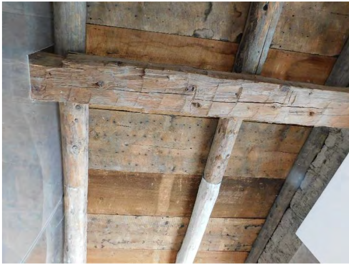
Ceiling within the public viewing enclosure. Note the original hand hewn wood beam, log purlins, and the wood board sheathing. Splices in the log purlins can be seen below center in the photograph.
