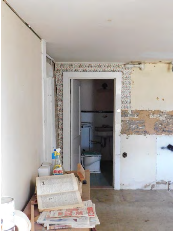
West end of the North wall; note variety of materials. Gypsum drywall ceiling was installed in the 1970's.
