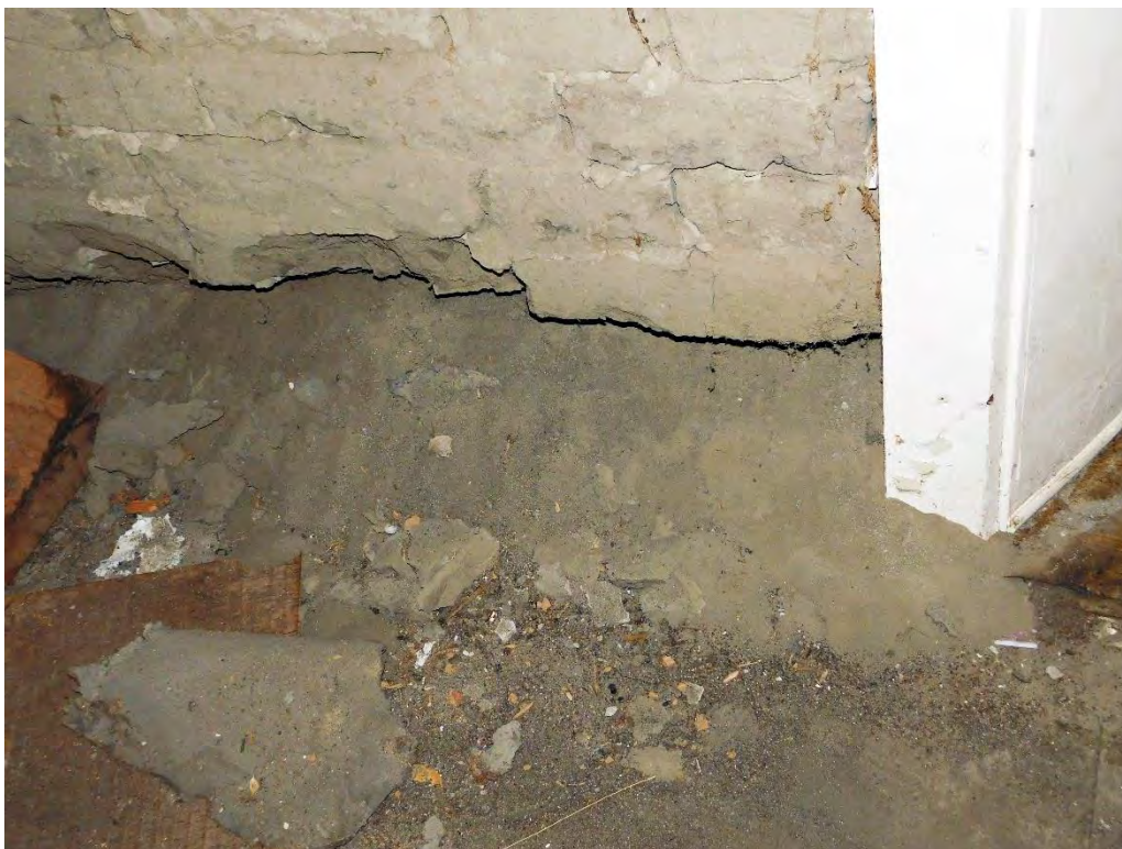
The adobe at the base of this wall exhibits substantial erosion. Refer to comments within the materials section of this HSR.
