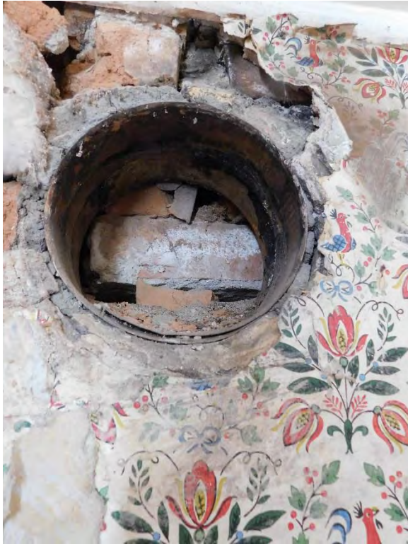
Thimble for stove located near the South end of the West wall of Room 104.
