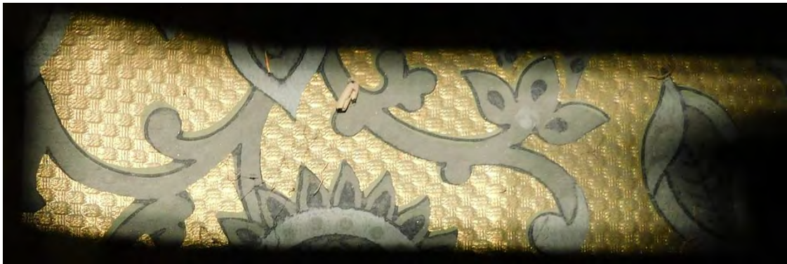
West wall of Kitchen / Utility 104. This wall was concealed by a newer furred wall and the wallpaper was found underneath. This is believed to be an 1876 wallpaper pattern.
