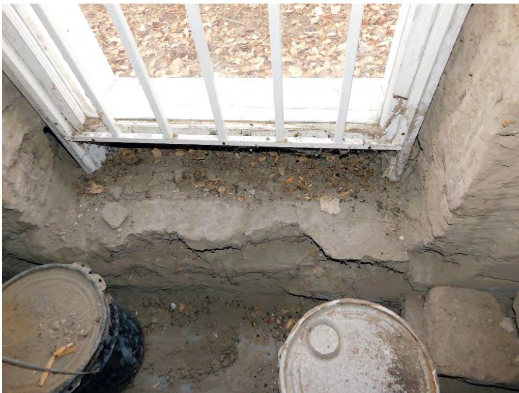
Window in the North wall; a contemporary metal security grille has been added. The adobe window sill exhibits damage.
