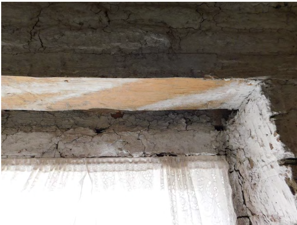
Window detail; note wooden lintel that supports the adobe wall.
