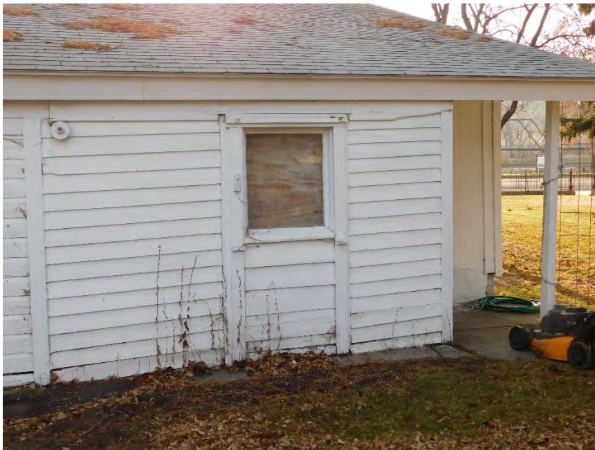
Southwest corner of the West Elevation. Note the use of corner boards, the different types of siding, and the splice location in the wall visible on the left side of the photo.
