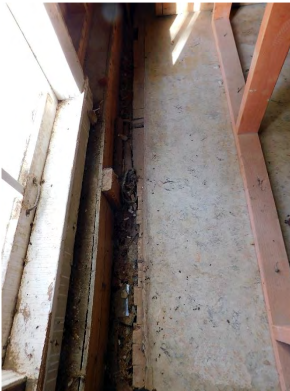
Looking down at base of South wall showing edge and forming of replacement concrete grade beam that supports new wood framed replacement wall. Note the ends of the original T&G fir flooring that can be seen on the right hand side of the gap.
