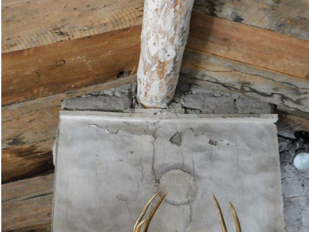
Top of fireplace chimney; note parging over adobe.
