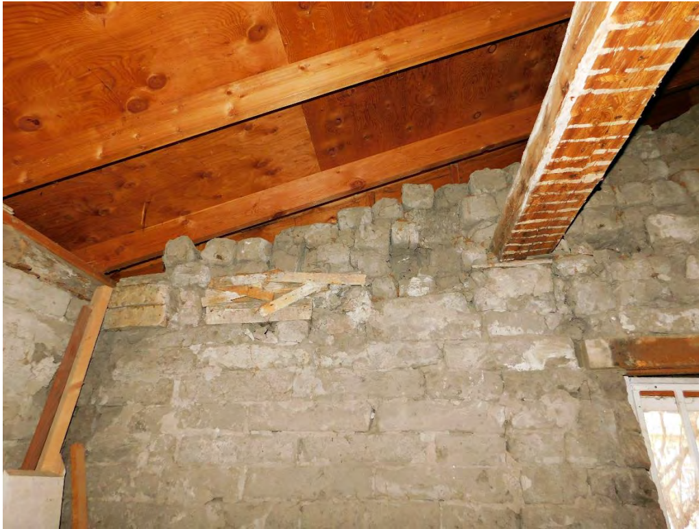
View of the upper part of the North wall; note the random size adobe blocks used to repair the top of the wall when the roof line was changed.
