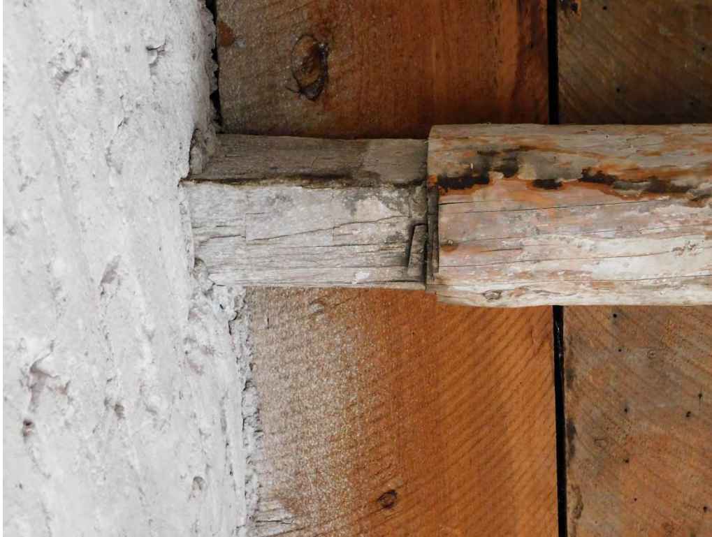
Detail of end of log purlin; note some of these purlins were re-set in the 1970's (see text)
