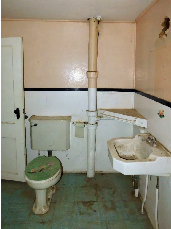
View of West Wall; flooring material is 8 x 8 tile that has been introduced into the historic residence in recent times.
