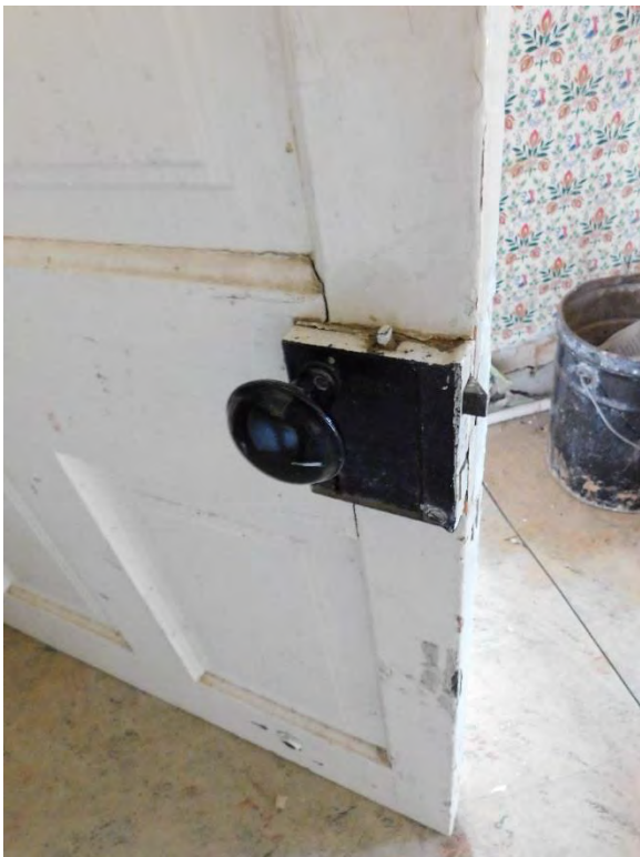
Surface mounted mortise lock on the door accessing the Kitchen / Dining area.
