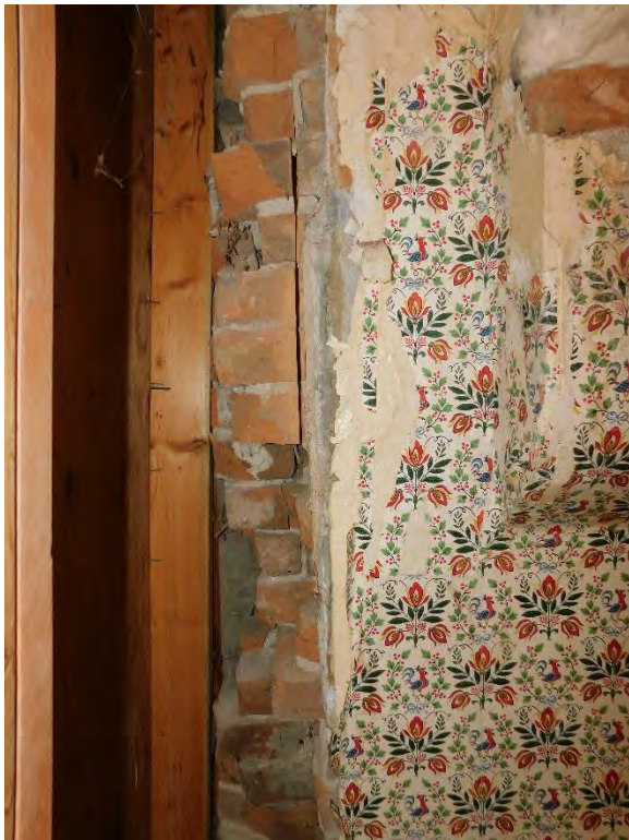
South end of West wall showing where original brick ends and replacement wood frame wall begins.
