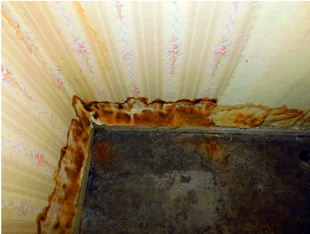
Close-up view of water damage. Note the wallpaper pattern.
