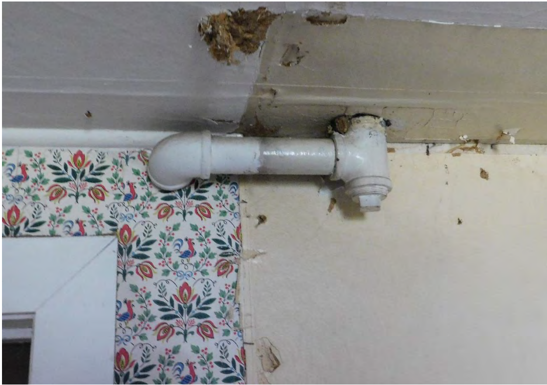
Intrusion from plumbing at ceiling along North wall of room.
