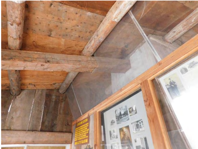
Ceiling detail showing the intersection of the 1970's plexiglass enclosure with the historic ceiling materials.
