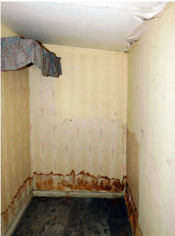
South end of Room 106. Damage from water is evident at the base of the wall.
