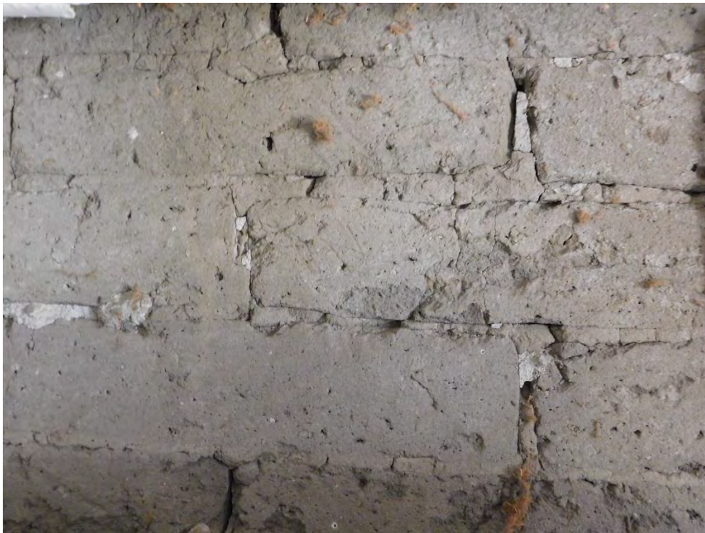
Detail of exposed adobe brick at the East wall of Room 104.
