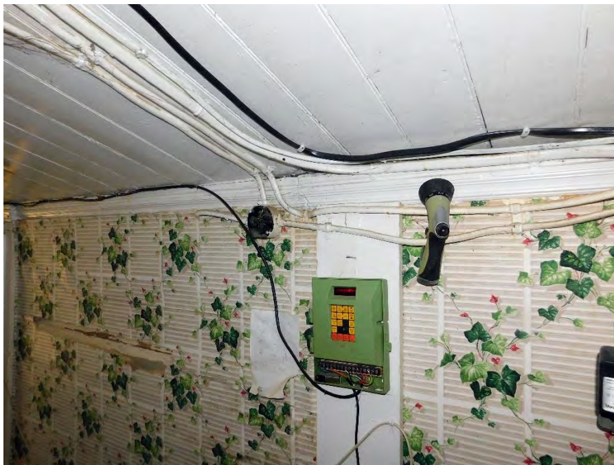
Irrigation controller located on the West wall of the rear vestibule. Note the various generations of exposed wiring.
