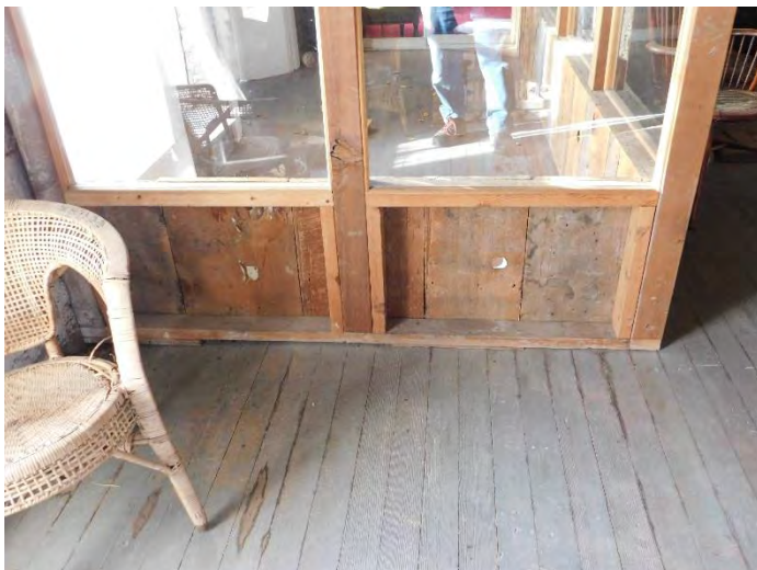
The T&G flooring from the North parlor continues on through to the viewing enclosure beyond. The wall construction and plexiglass relites are from the 1970's work.
