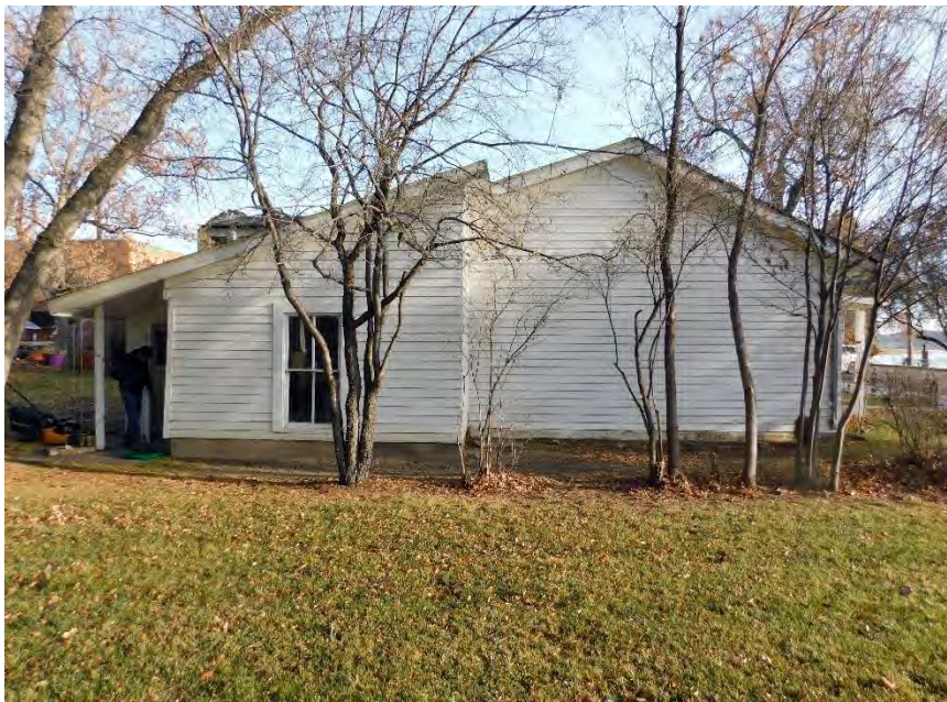
South Elevation. The window visible on this wall has been relocated; it originally was in the offset wall facing Front Street. Note that the chimney on this end wall has also been removed.
