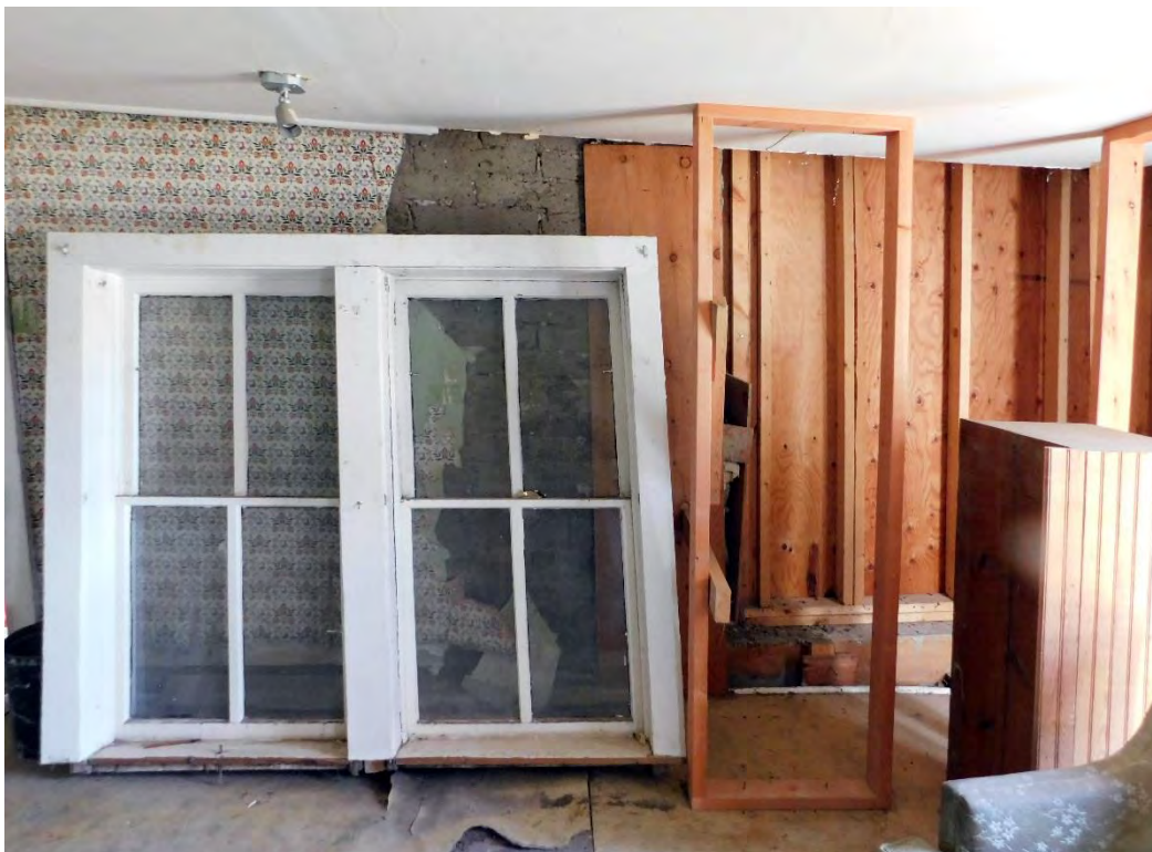
South end of East wall; the plywood indicates the location where the kitchen offsets past the plane of the South wall of the Parlor. The offset was originally built with brick walls but has been replaced with a wood frame wall in recent years.
